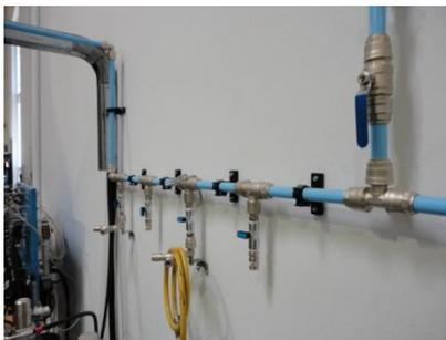
The flexible system design and color coding provided other benefits to Cefla. Using outlet/reducing tees close to point of use allowed for closely spaced outlets without condensate drop through, and the color coded tubing stands out cleanly against the white facility allowing the maintenance team to easily trace the air system. Cefla is so pleased with the aesthetics of the system that they will have Patton’s run it through their Café/showroom in the near future.
